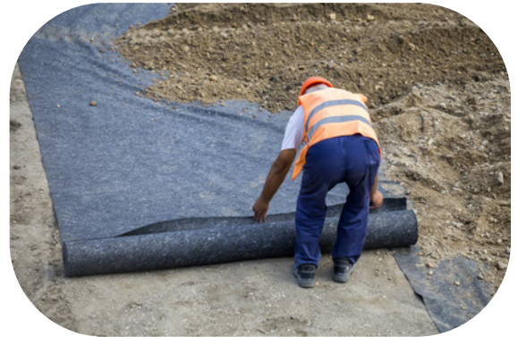
Worker laying geotextile in preparation for new building used for separation and reinforcement
