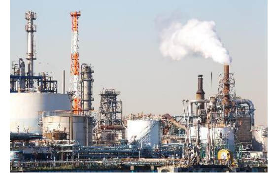
Industrial additives and by-products
